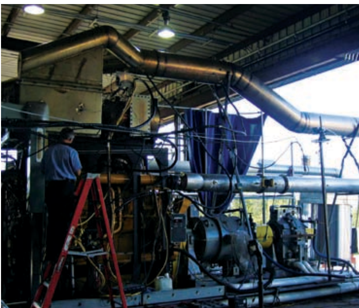
The SCR exhaust aftertreatment equipment that was developed by the manufacturer and SwRI engineers was implemented in a locomotive engine.
