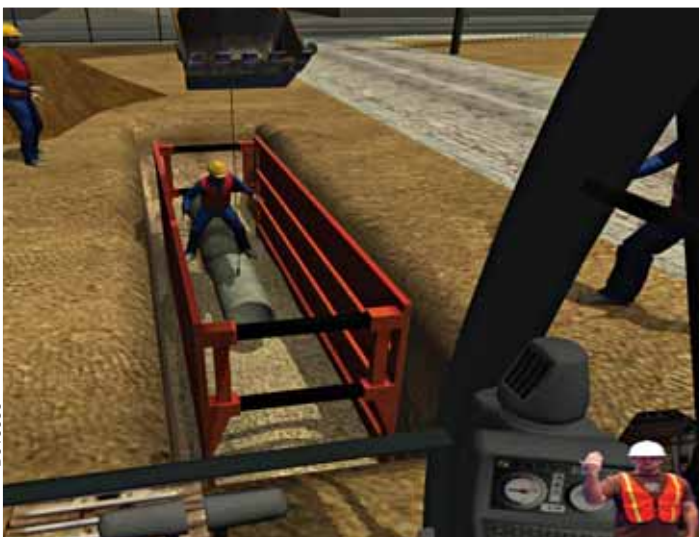
Trenching activity is simulated using SwRI-developed software that can train operators to excavate a trench, hoist and position a retaining structure inside it, and then operate the shovel within the workspace of the retaining structure, all without risk to personal safety.
