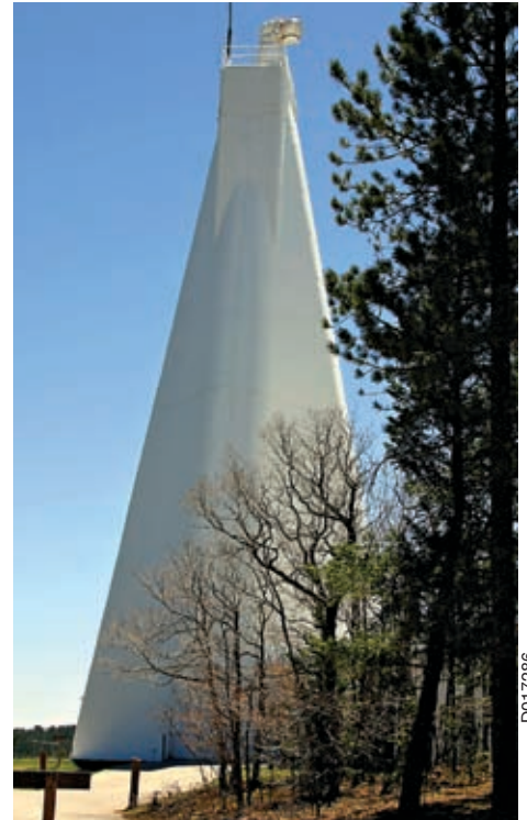
The SHAZAM instrument was recently deployed at the National Solar Observatory facility near Alamogordo, N.M. The telescope is more than 300 feet tall, with two-thirds of it underground.
