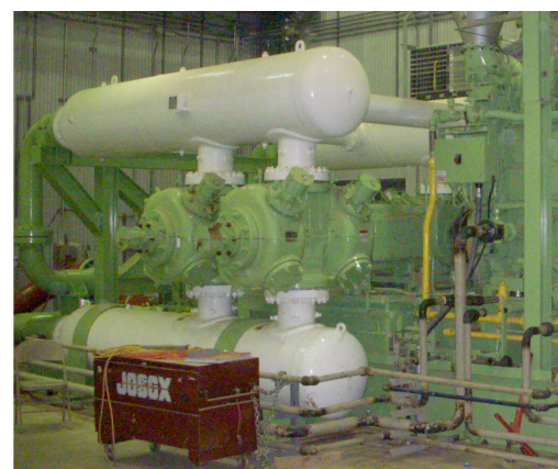
Figure 5. Field Site for Pulsation and Performance Testing of DDV Cylinder
