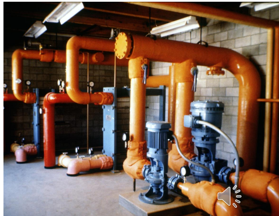
Heat exchangers and circulation pumps for the geothermal district heating system in Klamath Falls, OR. Photo courtesy Geo-Heat Center (NREL Pix 03694)
