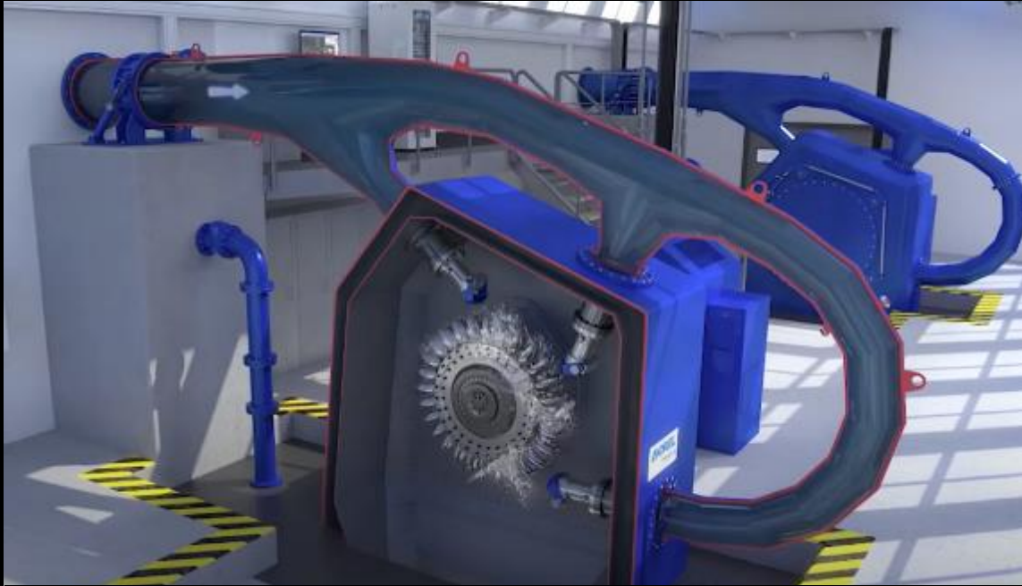
Sage's high-pressure Pelton turbine
