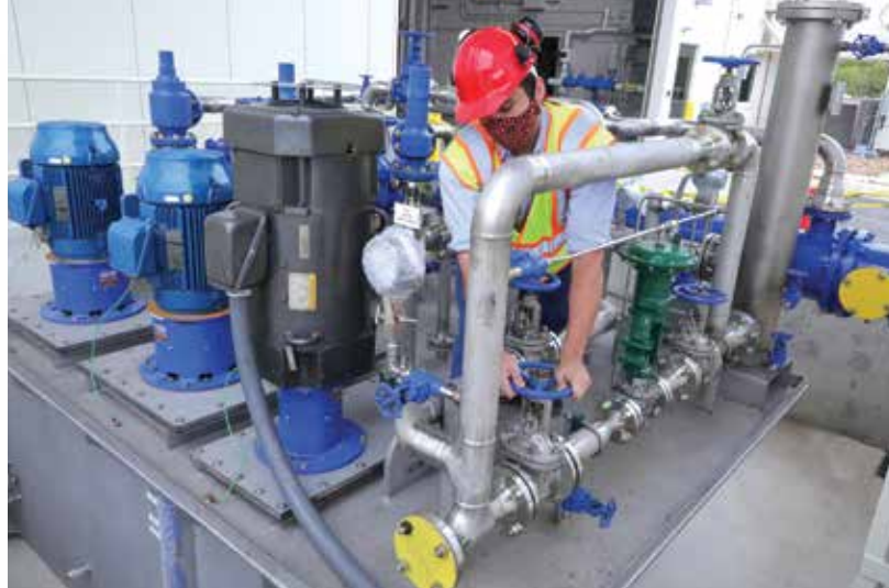
In 2020, SwRI completed construction of the STEP sCO 2 pilot plant building. We are now installing reconfigurable skid-mounted components, which allows the facility to evolve and keep pace with advancing technology.
