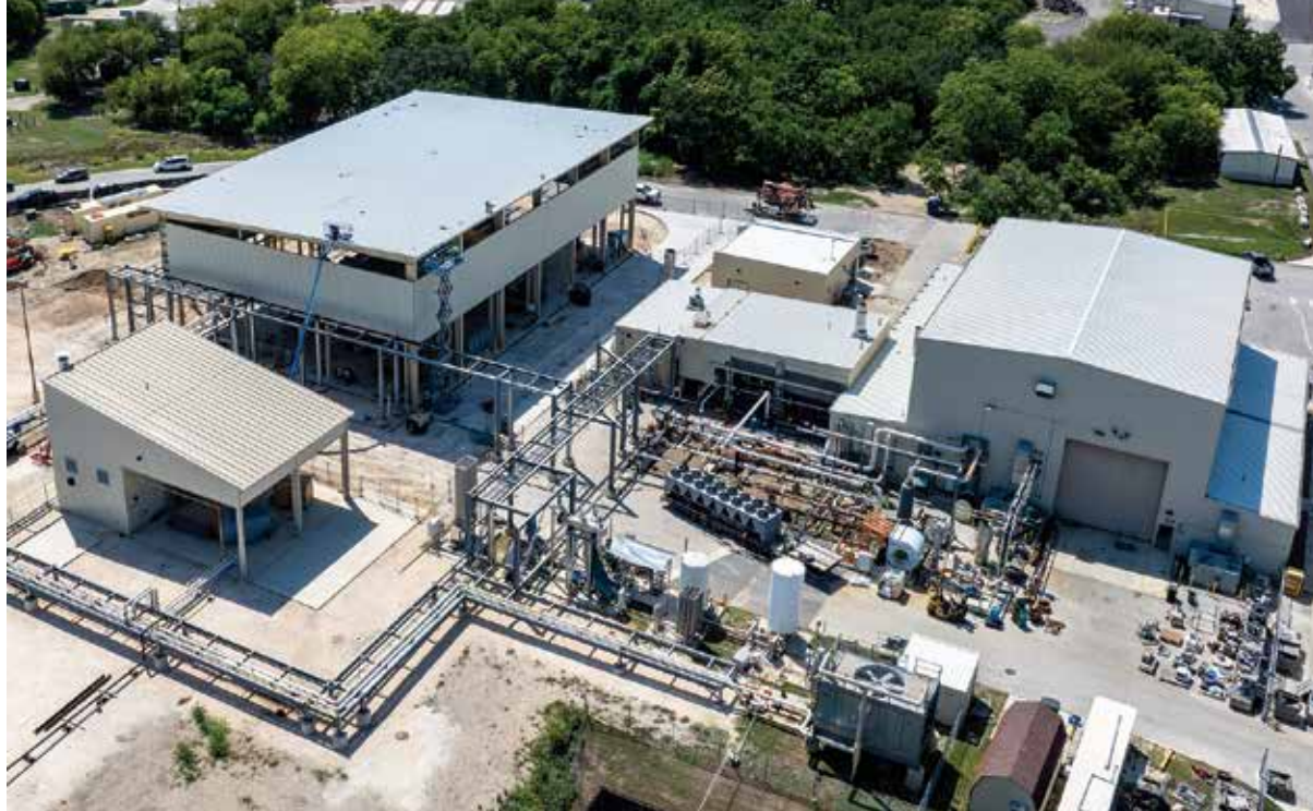
SwRI's new 90,000-square-foot Machinery Innovation Center for High-Energy Fluids offers megawatt-scale testing of machinery that operates with hydrocarbons and other flammable gases.
