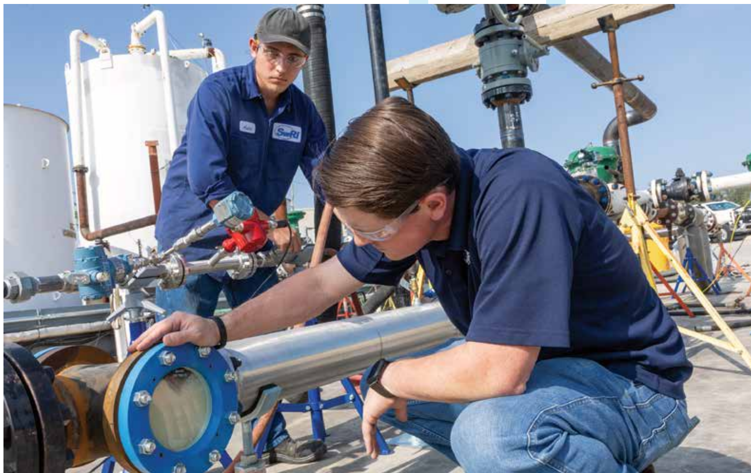
SwRI redesigned and optimized its HVFL, creating more permanent infrastructure to enable efficient cost-effective testing with heavy oils, including high-viscosity multiphase flows.
