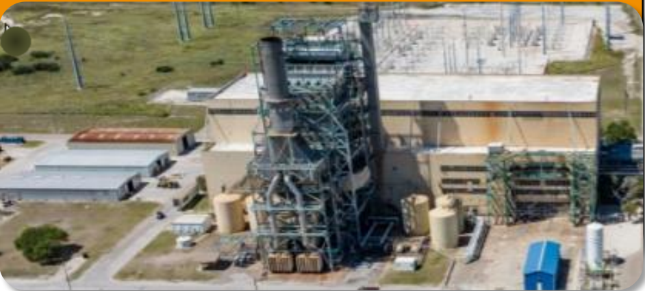
Barney Davis ST – 292 MW
