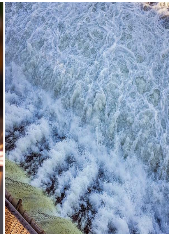
Water & Wastewater Treatment
