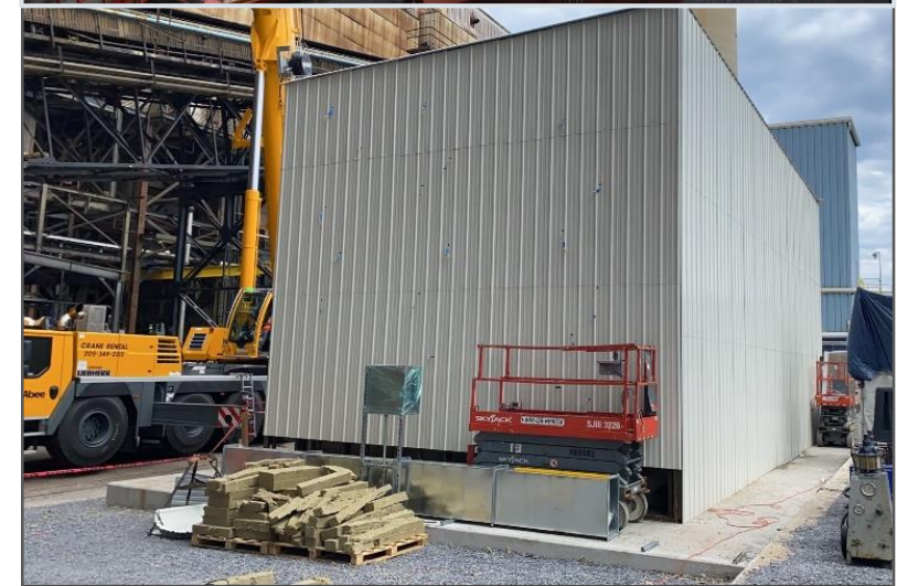
Gaston after installation of insulation and cladding
