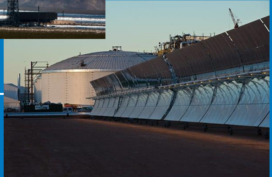
Solana CSP Plant in Arizona, courtesy Abengoa Solar Parabolic trough plant with 6-h storage → too expensive!
