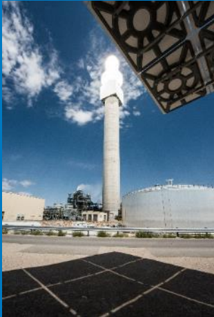
Last U.S. CSP plant was commissioned in 2015.
