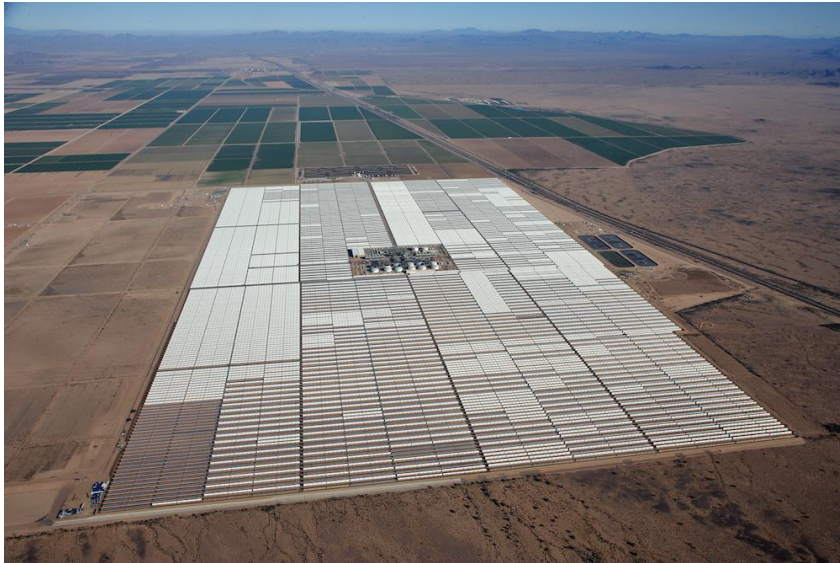
Solana's Mojave Solar Project (280 MW e )
