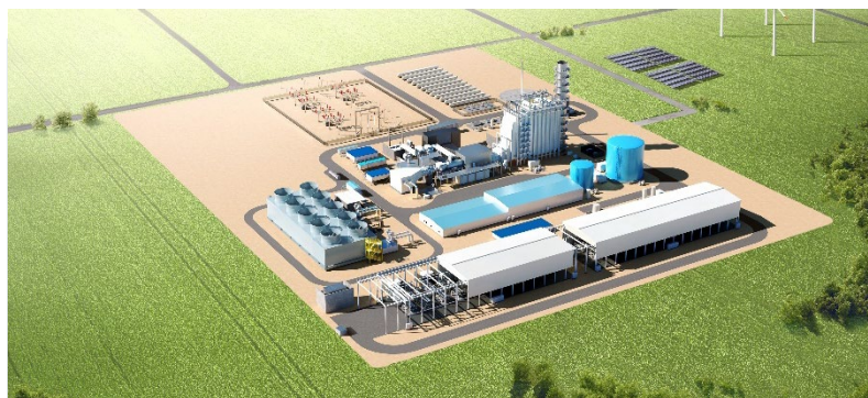
Hydaptive™ Integrated Plant: An all-in-one plant with hydrogen-capable power generation combined with a hydrogen production and storage facility
