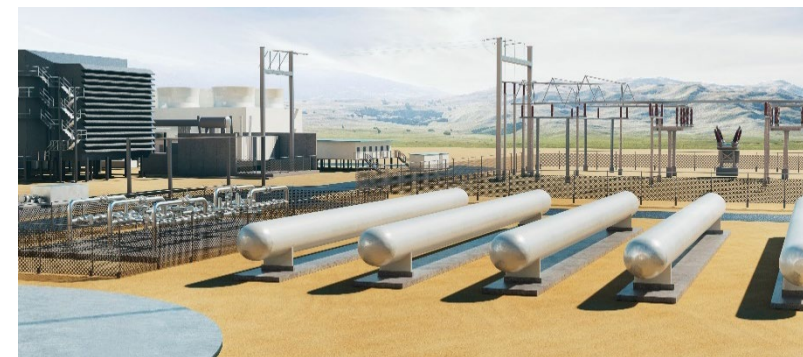
Hydaptive™ Storage: Standard hydrogen storage configurations can include a combination of pressure vessels and tanks, or geological structures such as salt caverns
