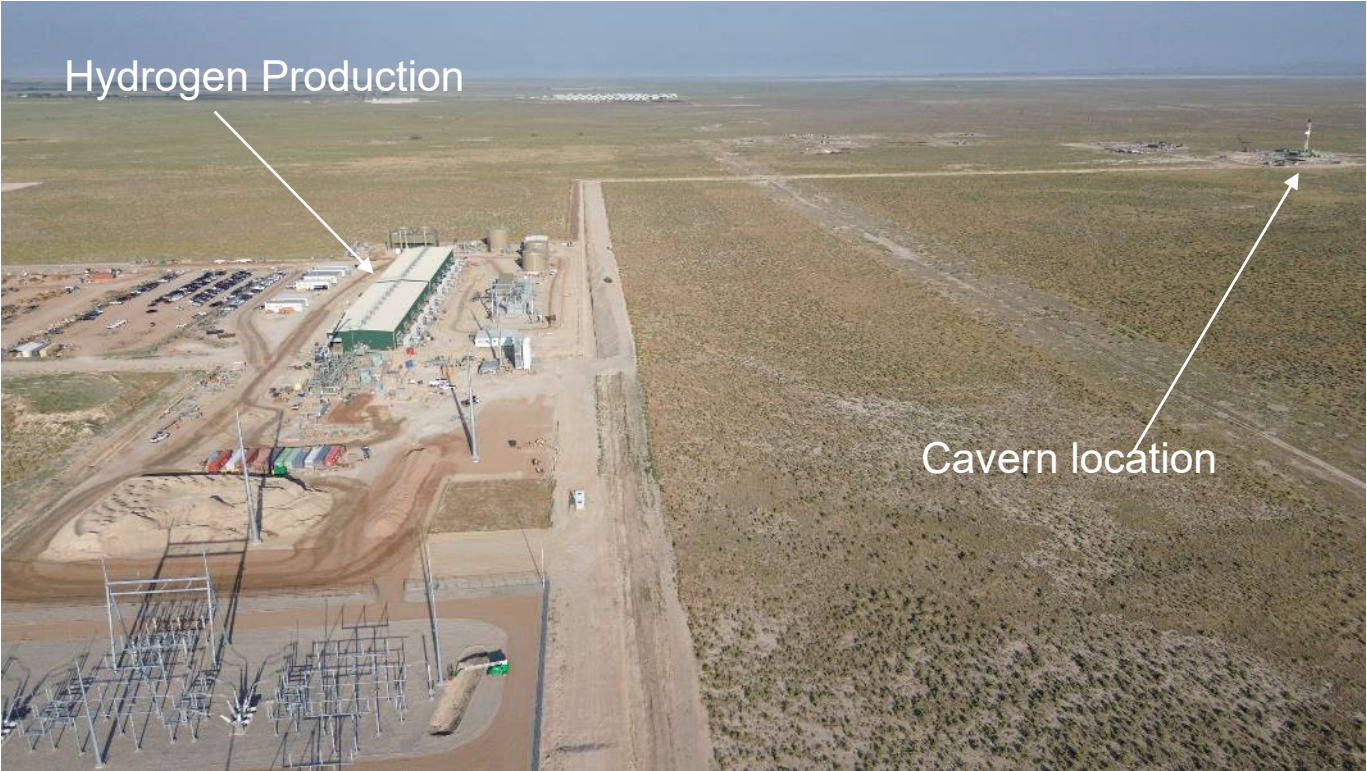
Empire State Building” sized cavern below ground...
